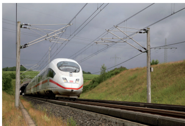
Fig. 1. ICE 3 and overhead contact line type Sicat H on the high-speed line Cologne – Frankfurt [Photo and Figures SPL Powerlines Germany]
