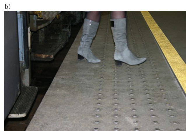
Fig. 7. Truncated domes within danger area at Warszawa Śródmieście railway station (a), direct exit from the carriage onto slippery truncated domes poses a threat for passengers (b) [Photo J. Poliński]
