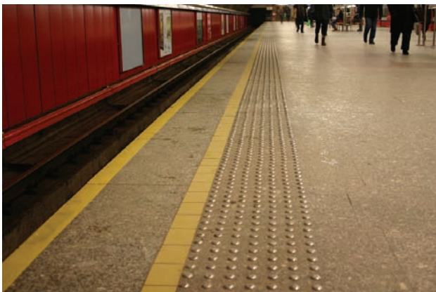
Fig. 2. View of marking on underground platform [Photo J. Poliński]
