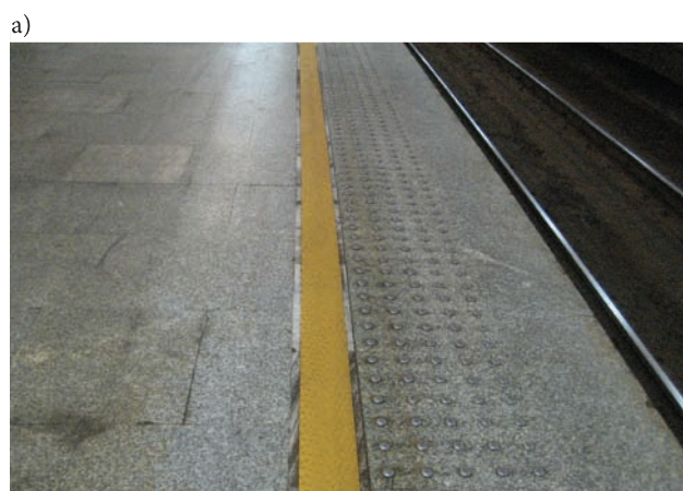
Fig. 7. Truncated domes within danger area at Warszawa Śródmieście railway station (a), direct exit from the carriage onto slippery truncated domes poses a threat for passengers (b) [Photo J. Poliński]
