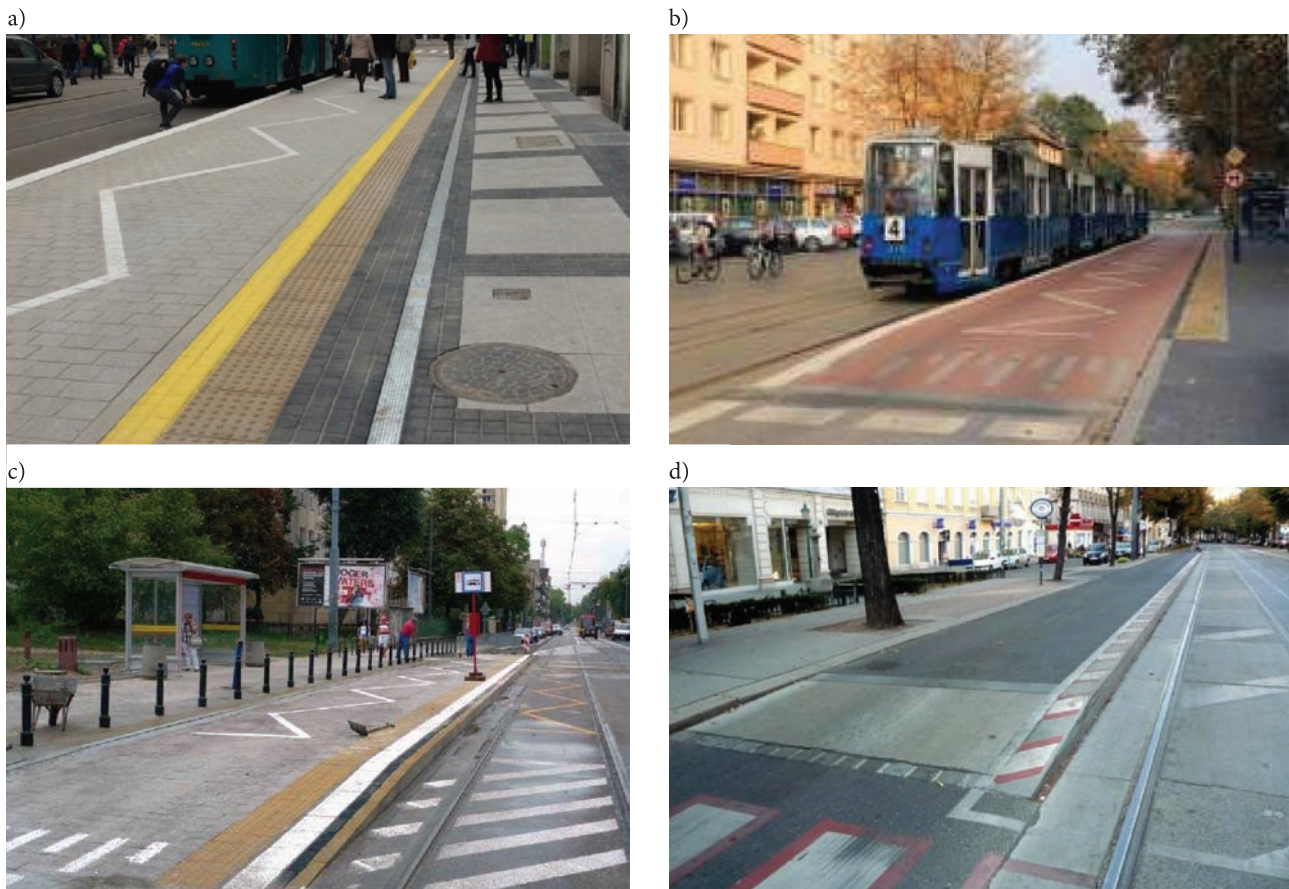
Fig. 5. Examples of tram platform Vienna style markings: a) Poznań [24], b) Kraków [25], c) Warszawa [26], d) Wrocław [27]
