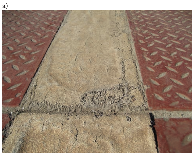
Fig. 6. Examples of platform tiles: a) damaged warning line on tiles without tactile elements, b) tactile warning surface placed on warning line [Photo J. Poliński]
