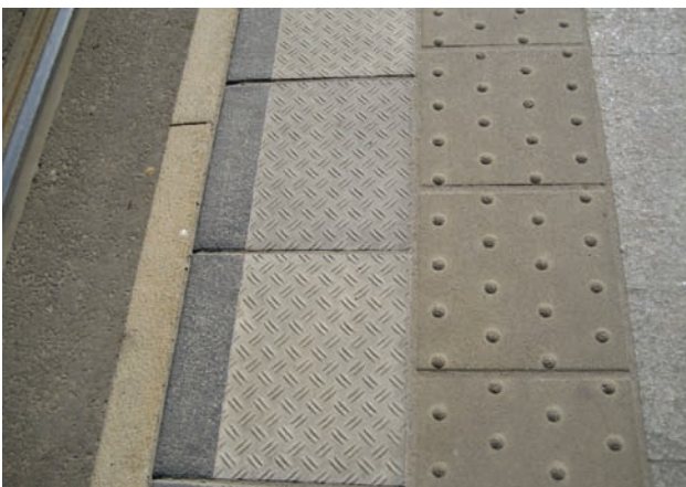
Fig. 9. Damaged corduroy bars in an underground passage under platforms at Warszawa Wschodnia railway station [Photo J. Poliński]
