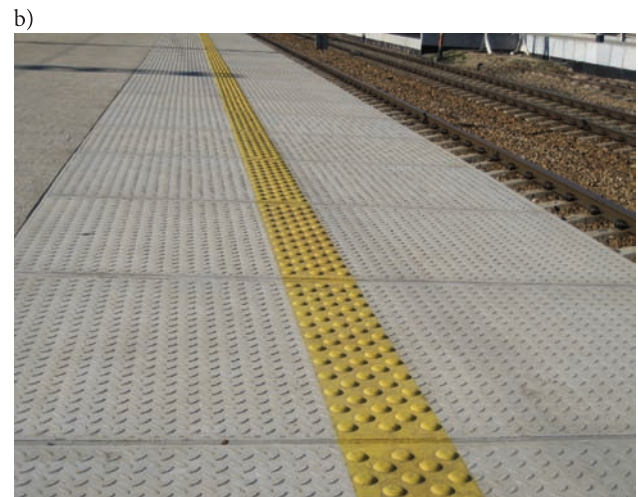
Fig. 6. Examples of platform tiles: a) damaged warning line on tiles without tactile elements, b) tactile warning surface placed on warning line [Photo J. Poliński]
