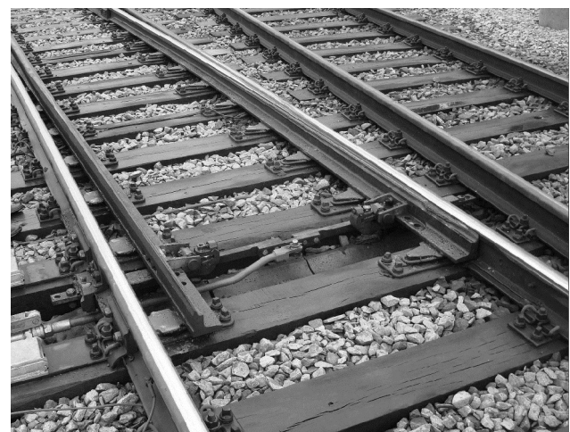
Fig. 2. Ordinary turnout switch panel [photo. M. Czarnecki]
