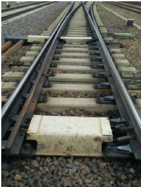
Fig. 1. Ordinary turnout with the angle 1:12 and arc radius 500 m [own picture]
