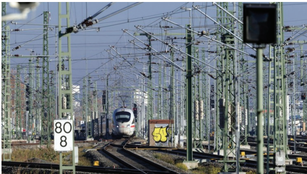
Fig. 2. With a developed railway infrastructure, it is easy to breach the structure gauge [3]
