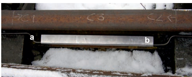
Fig. 5. Contactless heaters produced by TERMORAD, a) contactless heater, b) radiator [photo by D. Brodowski]
