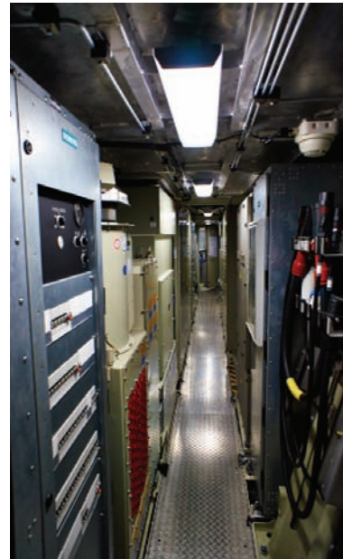
Fig. 10. Machine compartment of the Vectron locomotive [photo by Siemens]
