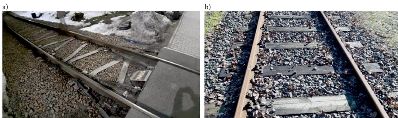
Fig. 1. Steel sleepers (a) and wooden sleepers (b) used in the construction of the railway track [photo D. Kowalczyk]
