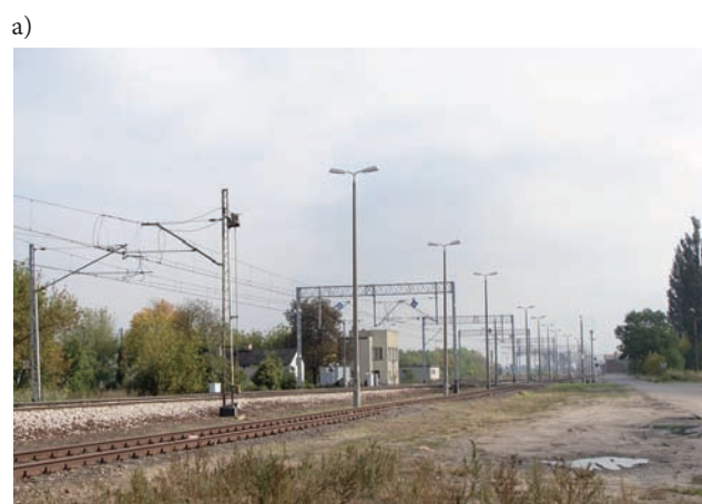
Fig. 5. (a) Sectioning of the YwsC120-2C type overhead contact line with a section insulator at a location where trains run with V max 160 km/h, no Y stitch wire at the insulator suspension point, Jackowice, 2012; (b) section insulator [photo taken by D. Dratwa]
