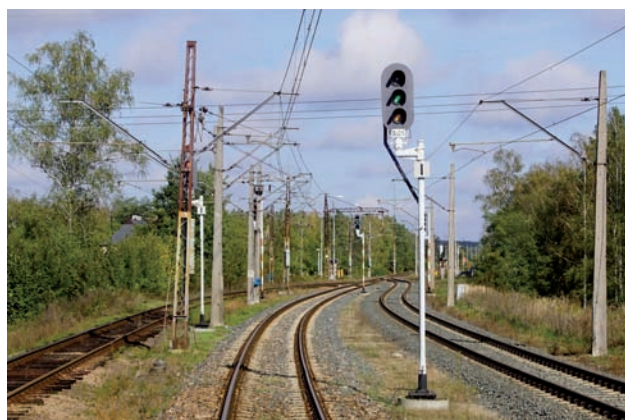
Fig. 14. Isolated tension span of an isolating switch No. 3 in a curve in Chociszew before station reconstruction, 2019 [photo taken by D. Dratwa]
