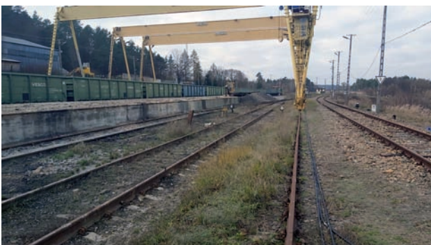
Fig. 23. Transshipment work at Werchrata Station (LK 101) (31 July 2021) [photo: J. Klimek / PLK]
