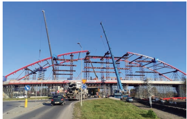
Fig. 16. Mielec – new road viaduct (3 December 2022) [photo: A. Stec / PLK]
