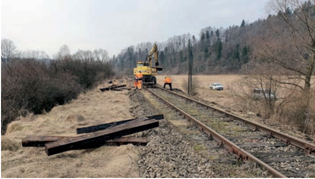
Fig. 22. Olszanica stop on LK 108 (26 March 2022) [photo: P. Hamarnik / PLK]
