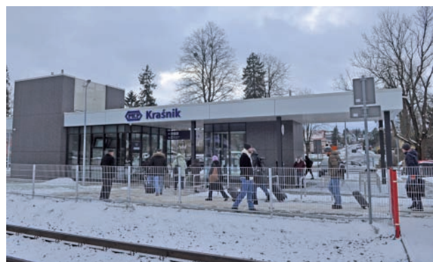
Fig. 11. The new station in Kraśnik, a so-called system railway station (24 December 2023) [photo by M. Graff]
