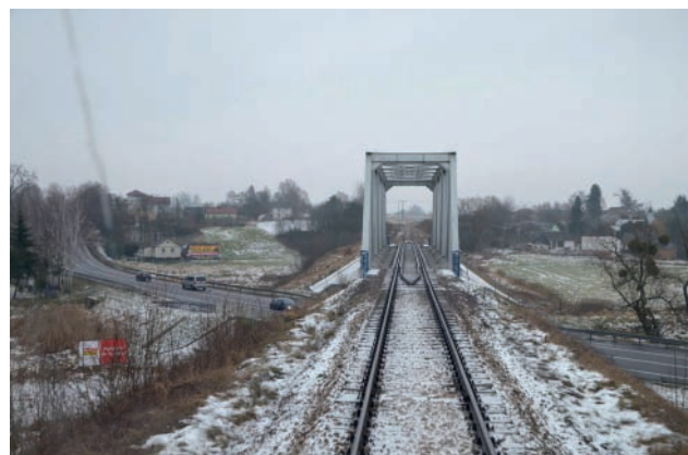
Fig. 22. The LK 68 before reconditioning; viaduct near Wilkołaz station [photo by PLK]
