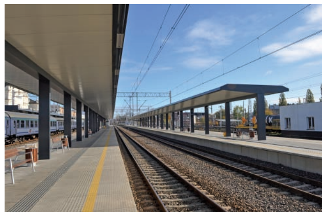
Fig. 6. Lublin station after reconditioning (23 October 2021) [photo by M. Graff]
