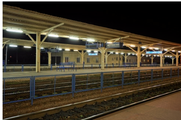
Fig. 5. Lublin station before reconditioning (25 October 2014) [photo by M. Graff]
