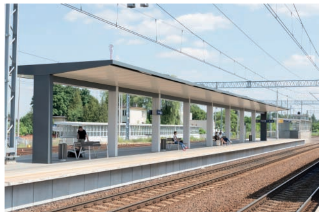
Fig. 8. Dęblin station after reconditioning [photo by G. Biega/PLK]
