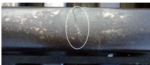
Fig. 3. Rail squat defect [photo by I. Mikłaszewicz]
