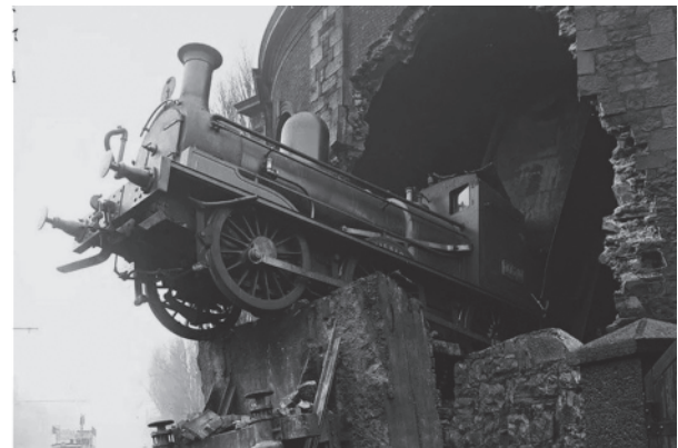
Fig. 2. Derailment of a train at a station in Dublin, Ireland, in 1900; a fragment of the track end device can be seen beneath the locomotive; National Library of Ireland [8]
