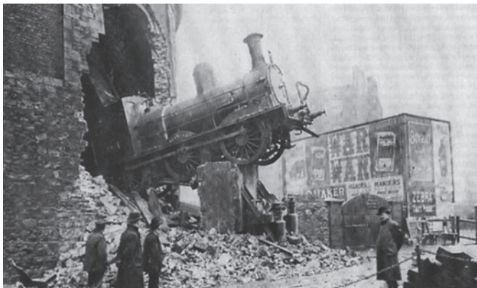
Fig. 2. Derailment of a train at a station in Dublin, Ireland, in 1900; a fragment of the track end device can be seen beneath the locomotive; National Library of Ireland [8]
