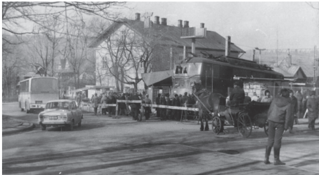
Fig. 4. Train derailment at Zakopane Station (23 March 1979); the locomotive failed to stop within the station tracks, destroyed the buffer stop, and ended up on Kościuszki Street [7]
