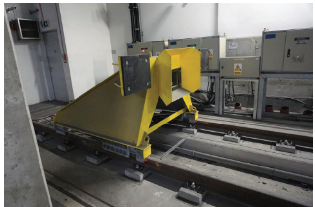
Fig. 11. Sliding buffer stop – Metro M2 [photo by D. Kowalczyk]
