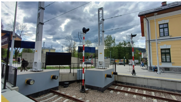
Fig. 5. Zakopane Station – terminal station, current solutions for track end devices (17 May 2024) [photo by W. Kowalczyk]
