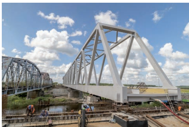
Fig. 7. Uhowo on LK 6 (156.265 km mark), construction of a new bridge over the Narew River [photo by Ł. Brylowski/PLK]
