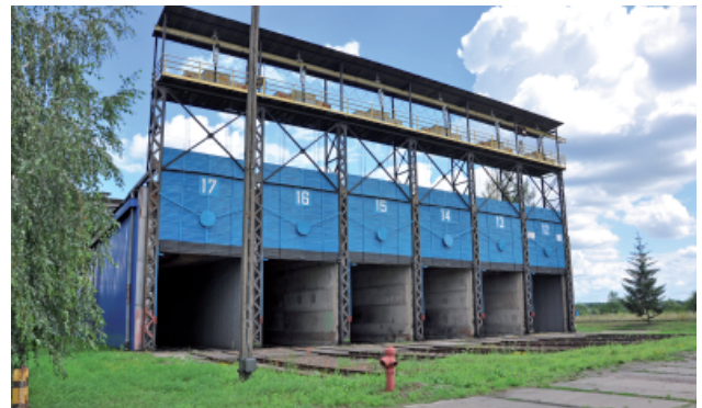
Fig. 13. Iron ore thawing facility at Medyka station (28 July 2015) [photo: M. Graff]
