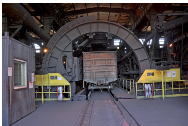
Fig. 18. Hall equipped with wagon tipplers for unloading iron ore at the Katowice Steelworks Ore Transshipment Base, Dąbrowa Górnicza / ArcelorMittal Poland (25 June 2016) [photo: M. Graff]
