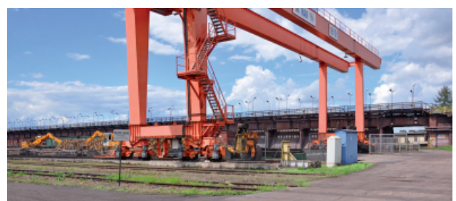
Fig. 16. Station for the gravity unloading of iron ore at Medyka station (28 July 2015) [photo: M. Graff]
