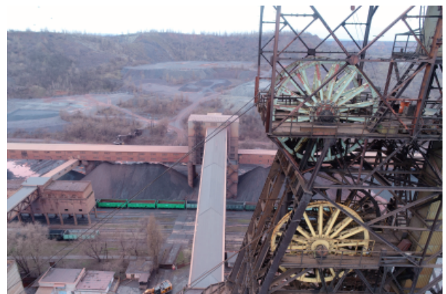
Fig. 24. Frunze underground iron ore mine, Kryvyi Rih, Ukraine (19.12.2017) [photo: Sukhabalka / Wikimedia Commons]
